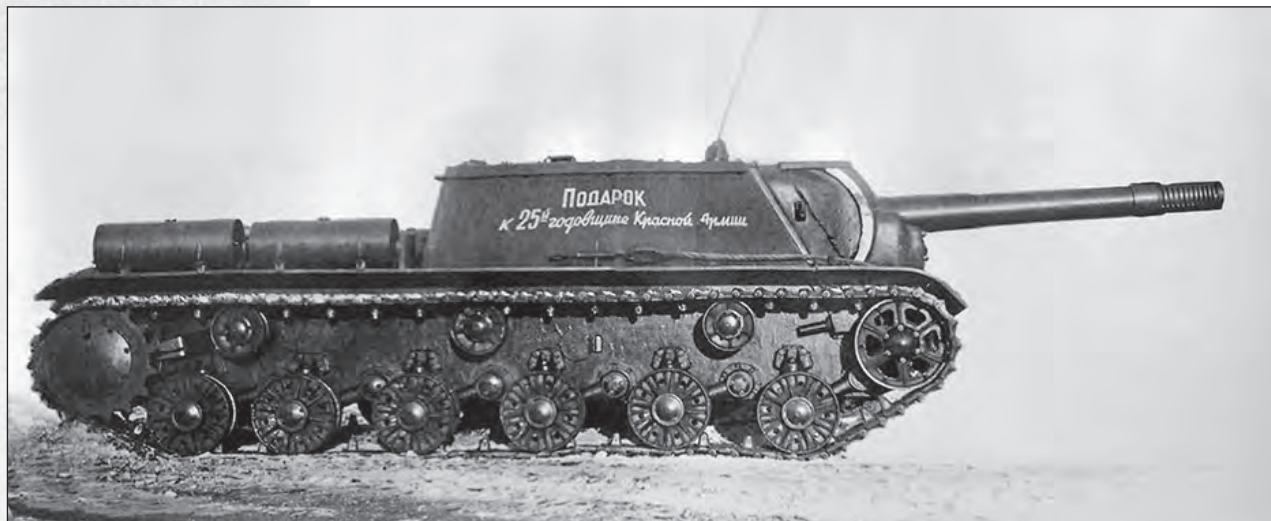
Right side view of the KV-14 prototype. Construction of the SP gun was set for February 23 (TsAMO).
